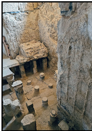
Sub floor of bath house
