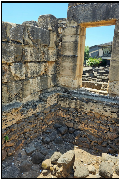
Foundation of 1 st C. Synagogue
